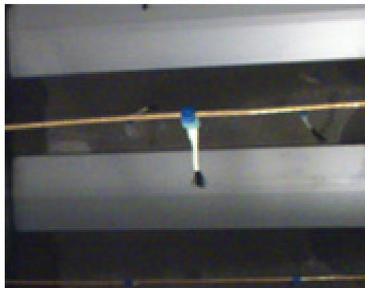
**Figure 3.** Photo of one ionizer brush mounted in an air handling unit..
